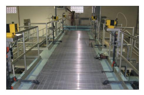
The D2 System is available as above ground stainless steel package units or, for larger flows, multiple 50 square foot modules are installed in concrete tanks. The internals are shipped in easy-to-assemble sections and field assembled. Advanced SCADA controls are normally supplied as part of the system design.
