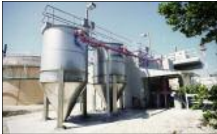
DynaSand Filter above ground package units
