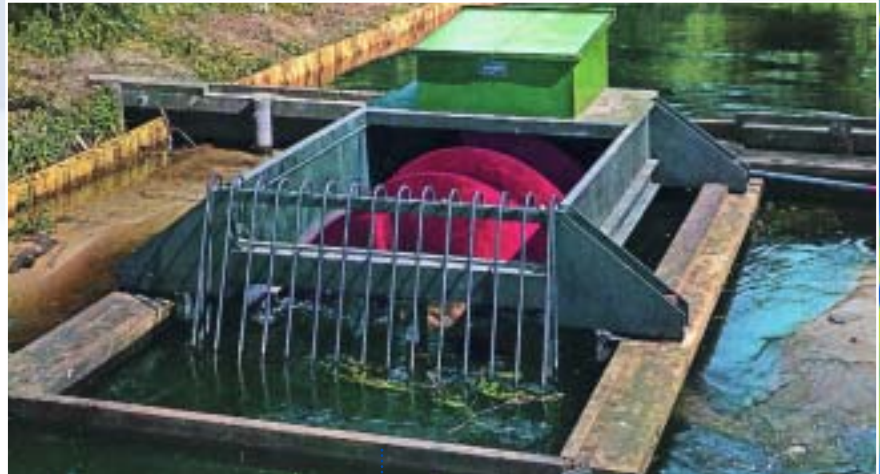
Horizontal Flushing Installation
