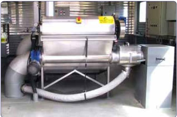
Prior to installing a Salsnes Filter system, the Enderby WWTP produced sludge with only 1- 2% DM. Installing Salsnes upstream of the oxidation ditch reduced the plant's total sludge volume by 87% - thanks to the integrated thickening and dewatering processes in the Salsnes Filter SF:4000.
