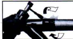
**3** Heat Shrink Sleeve with wide billowy flame. **Do Not Use Pin Point Flame.** Work flame around joint evenly.
