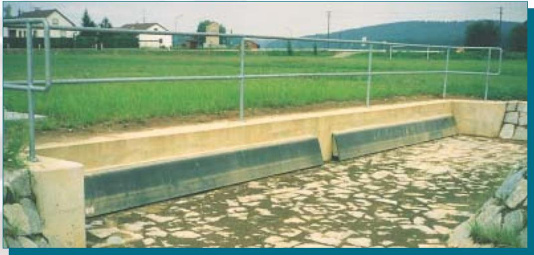
Typical installation: The **ACU-FLAP** Check Elements at overflow structure.
