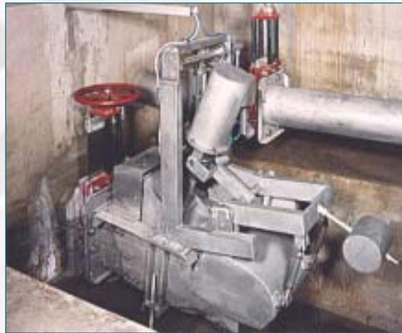
ACU-JET flow regulator with servo-control system
